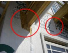
The firestopping should be improved around the A/C freon lines and gas line in the sole plate between the top floor and the attic as to the IRC. See photo.
