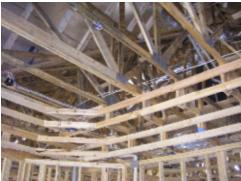
TeckShield decking has been installed throughout the attic. I have attached a web site that will address this products and the benefits. <a href="http://www.lpcorp.com/radiantbarrier/radiantbarrier.aspx">http://www.lpcorp.com/radiantbarrier/radiantbarrier.aspx</a>>
