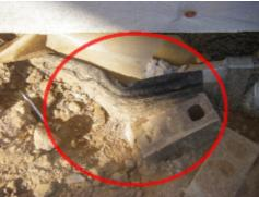
The vapor barrier, house wrap is damaged along the front and should be repaired.
