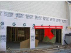
The footing drain along the right side of the home should be protected against damage. Currently, the drain is crimped and is above grade.
